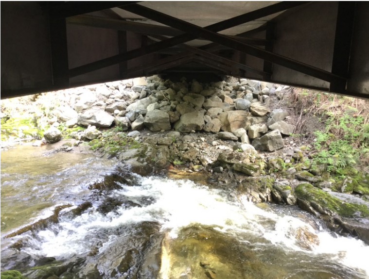
Left Bank Abutment when facing downstream
