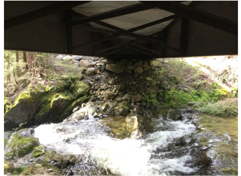
Right Bank Abutment when facing downstream
